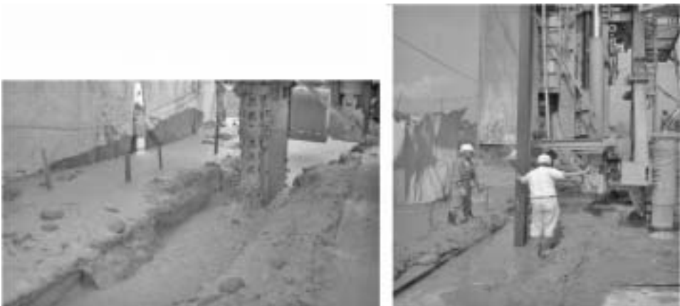
(a) (b) Figure 13 Trial wall excavation using air foam suspension
